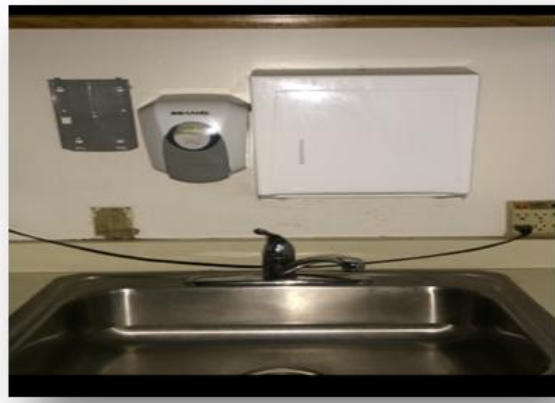
AFTER – Service Area Kitchen Sink Area
