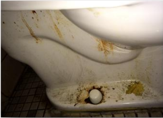
BEFORE – Service Area Restroom Toilet 2
