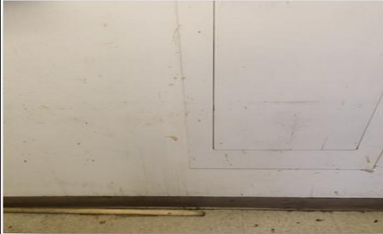
BEFORE –Service Kitchen Walls
