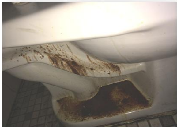
BEFORE – Service Area Restroom Toilet 1
