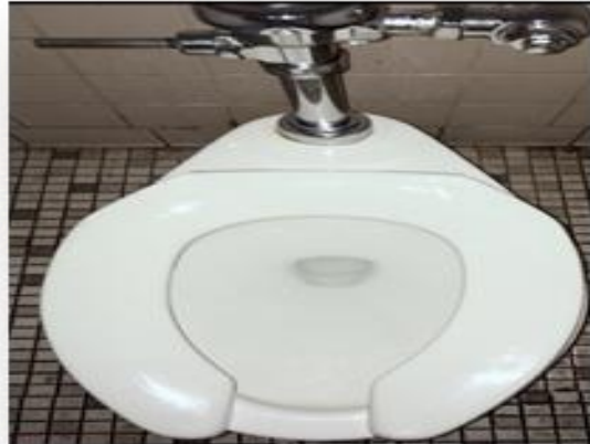
AFTER – Service Restroom Toilet 1
