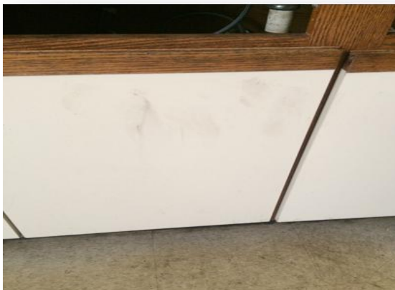
BEFORE –Service Area Kitchen Cabinets
