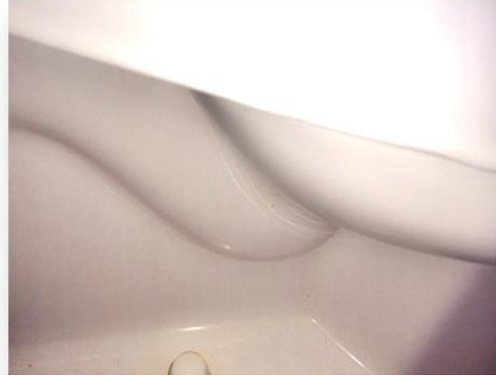
AFTER – Service Restroom Toilet 2
